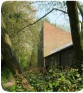
Central part of Ash House
